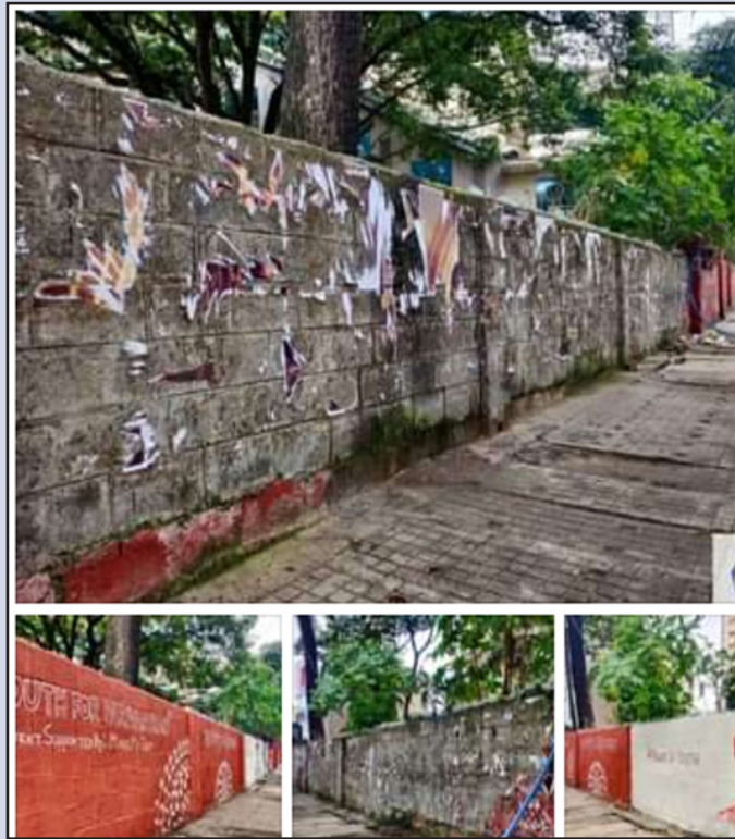
Students from 8th semester involved themselves in cleaning the roads and painting the road side walls at sarakki signal on Dr.Puneeth Rajkumar road.
